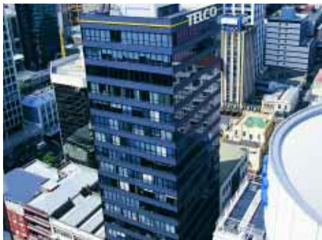
The Telco Building
