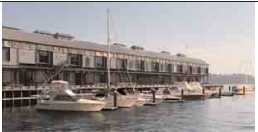
Walsh Bay Moorings Pier 8/9, Sydney
