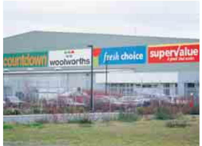
Christchurch Distribution Centre
