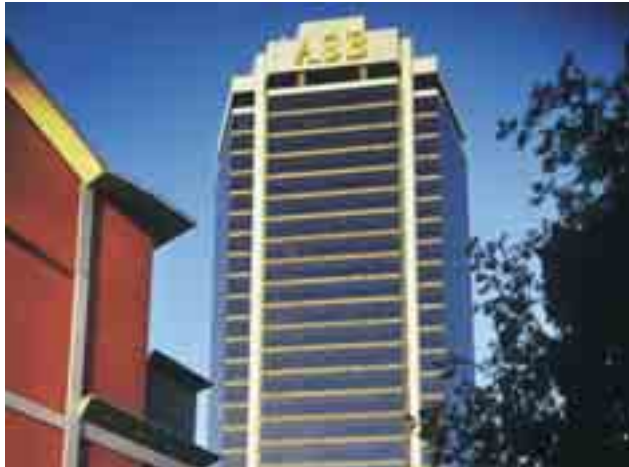
ASB Bank Centre
