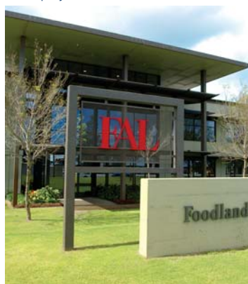
FAL Property Trust - Foodland Distribution Centre
