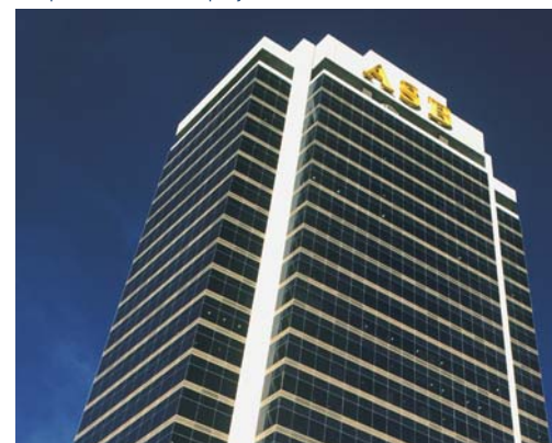
Multiplex New Zealand Property Fund - ASB Bank Centre
