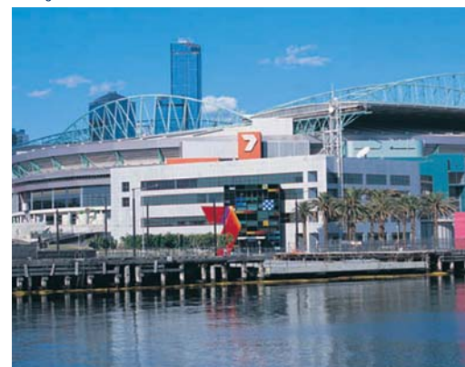
Trafalgar Platinum Fund No. 12 - Melbourne Broadcast Centre
