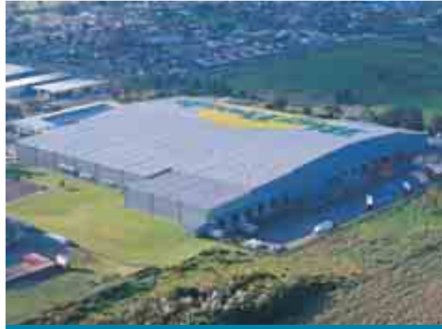
Wiri Distribution Centre
