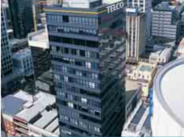
The Telco Building
